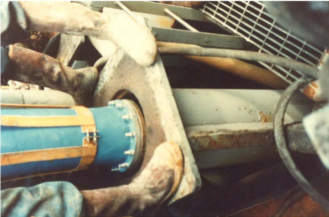
**Figure 3. FIBERBOND(R) column pipe section set into steel casing.**
